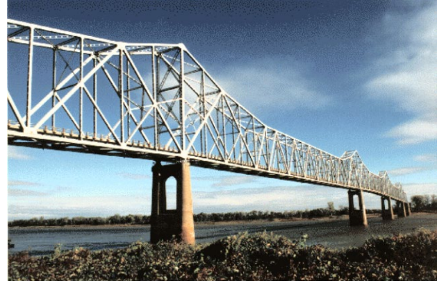
(b) US51 Bridge
