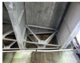
(b) Main girder end
