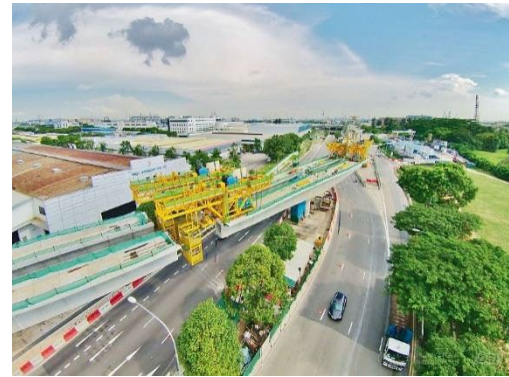
Fig. 2(b). Balanced Cantilever using Lifting Frames
