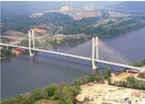
(c) Maysville Bridge
