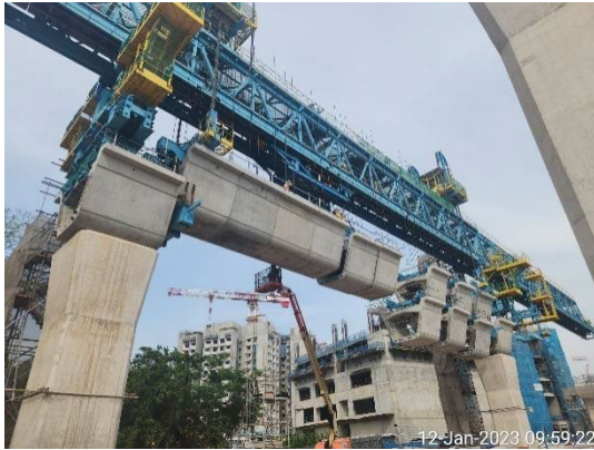
Fig. 2(a). Segmental Launching using Lifting Girder
