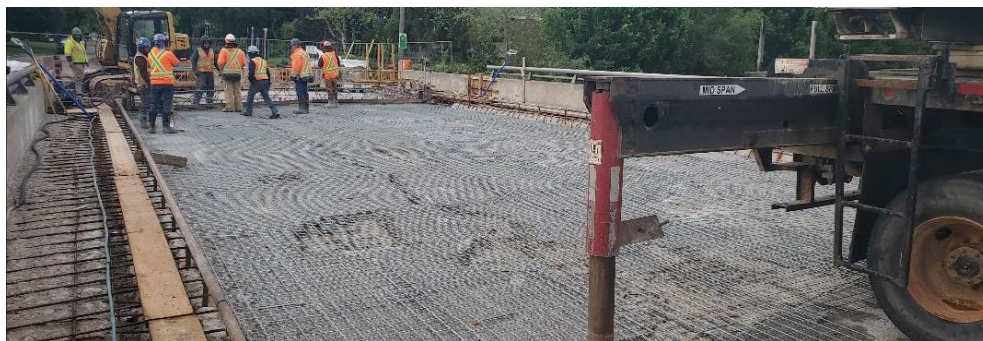
Fig. 4. Curry Avenue Surface Preparation
