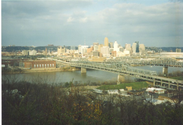
(a) Brent-Spence Double Deck Bridge
