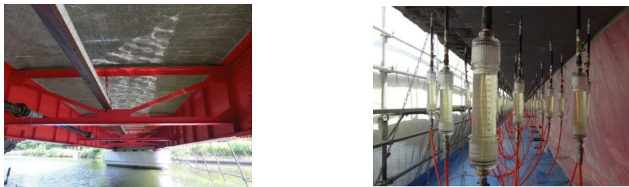
Fig. 6. Lithium pressurized injection from underneath the deck
