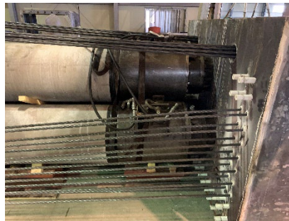
Fig. 5. Arrangement of internal reaction arm (PHC piles) and an anchoring block
