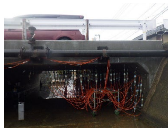
Fig. 7. Maintenance work without traffic regulation
