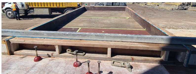
Fig. 1. Form for the Dura ® ECC Trial Batch
